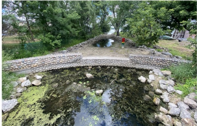
The headwaters of Bassett Creek at Medicine Lake. When water levels are high, the creek spills over the concrete weir.
