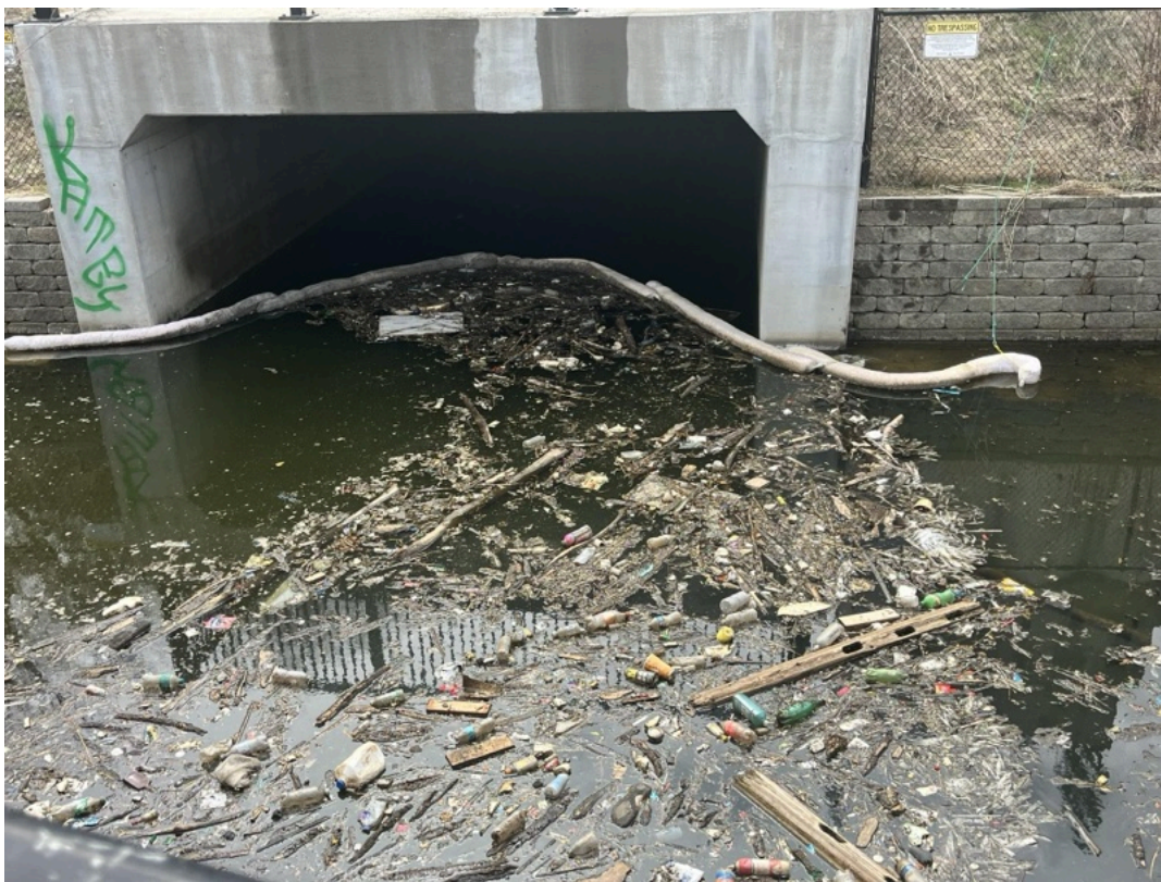
Bassett Creek New Tunnel Outlet April 2026
